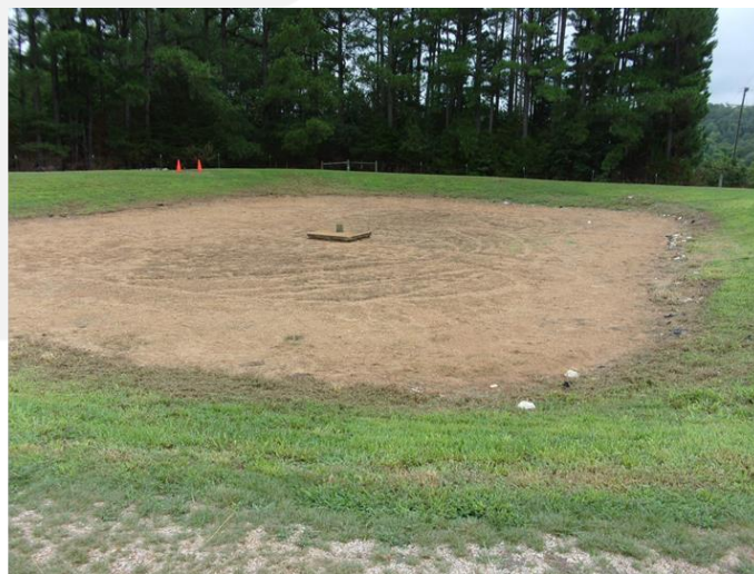
After – Sand filter clear of vegetation
