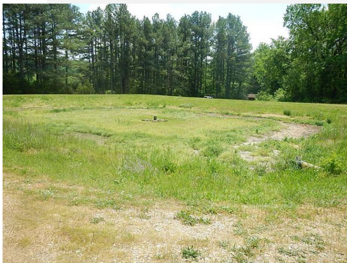
Before – Vegetation overgrowth in sand filter
